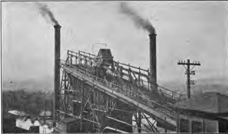
SKIP DUMPING AT No. 1 TIPPLE SHOWING ARRANGEMENT FOR DUMPING EITHER ORE OR POOR ROCK—RAIMUND
